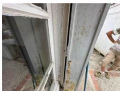
Joint menuiseries séjour
